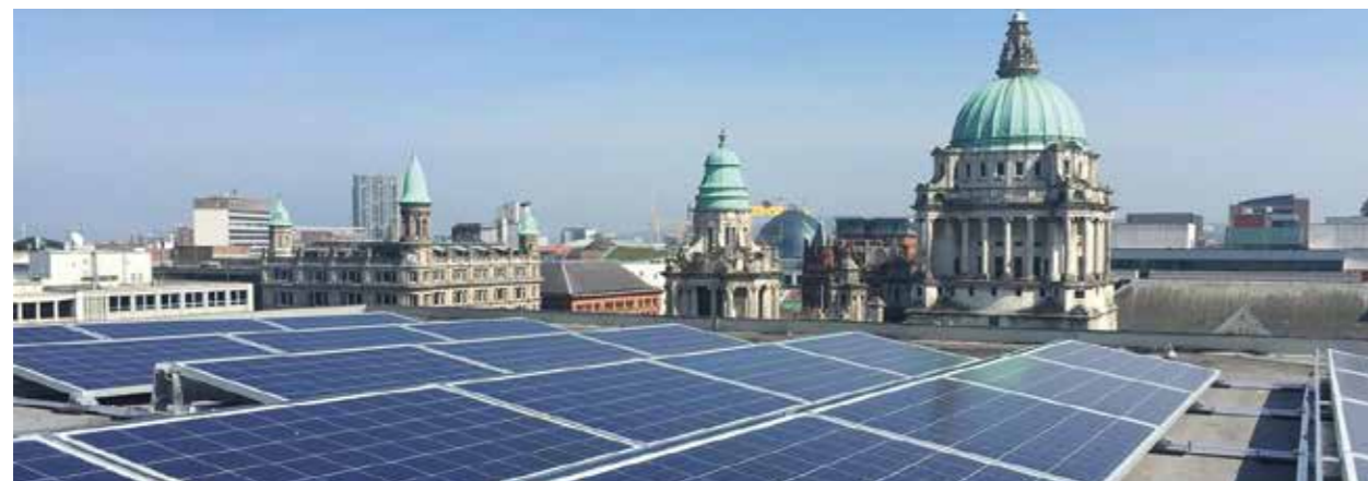
Solar panels on our head office at Donegall Square West, Belfast.
