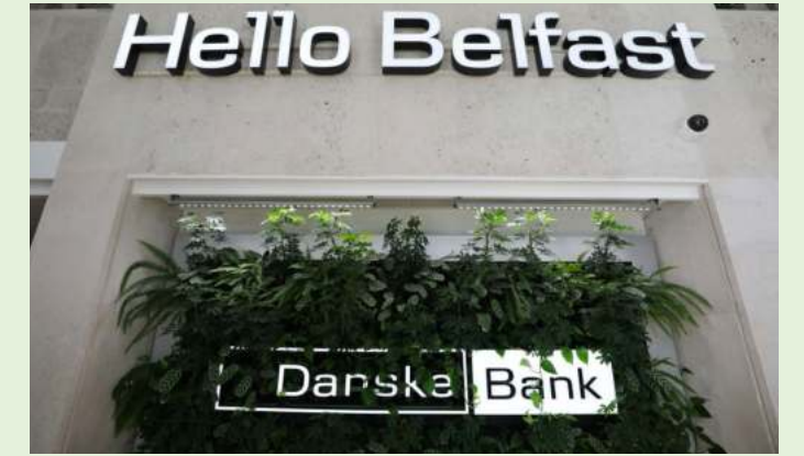
Donegall Square West branch in 2024 with its green 'living wall' (a nod to the bank's growing focus on supporting the climate change agenda).
