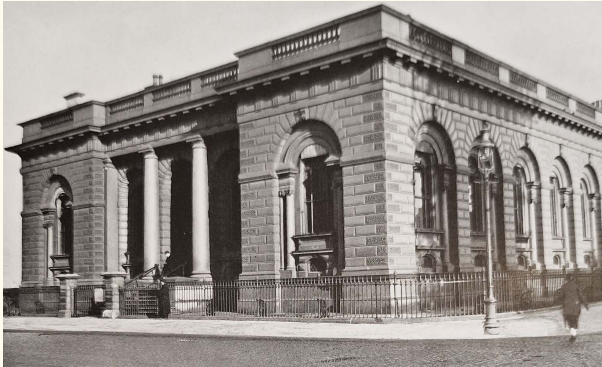
Sir Charles Lanyon's magnificent head office building, built in 1852.
