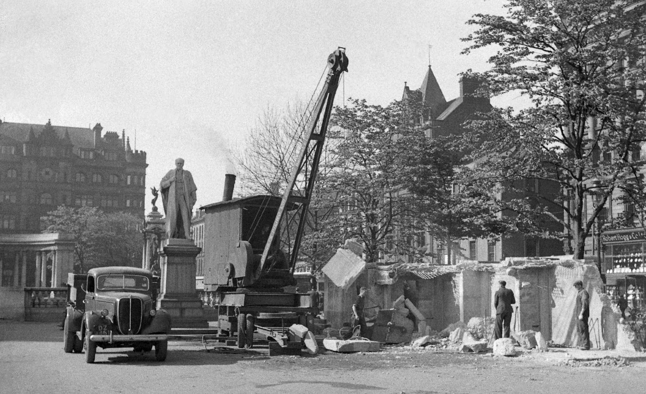
Taking down the air raid shelters in the City Hall grounds Belfast, 2 May 1945.
